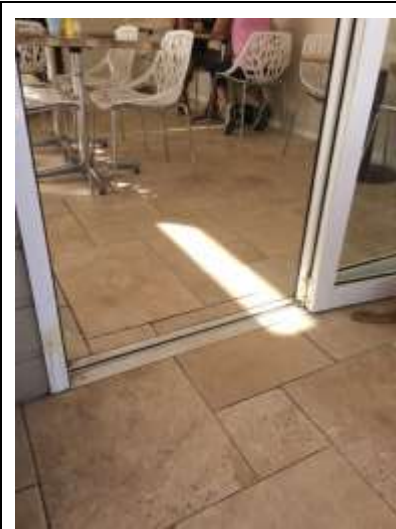
Figure 12 – Photograph of door threshold
