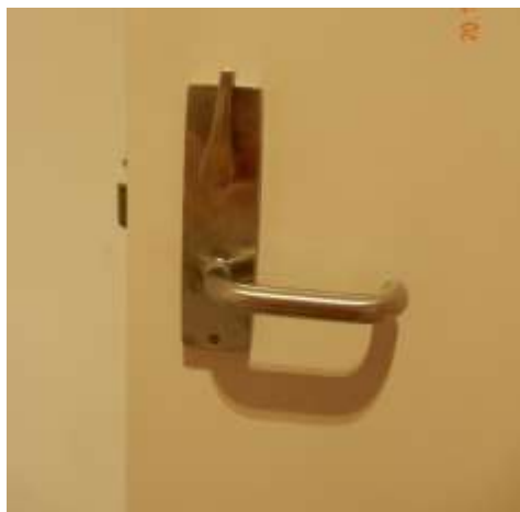
The above image indicates a privacy latch set provided to accessible WC facilities as viewed from within the facility
